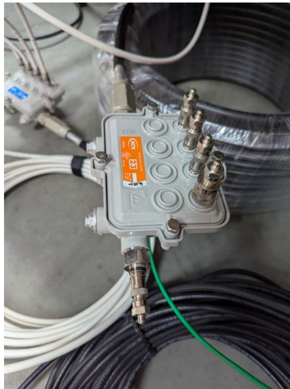
Figure 7 – Second Tap Terminated
